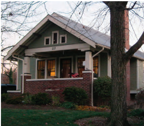
Porch Detailing and Exposed Beam and Rafters
