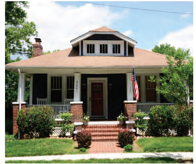
Brick Pier Column Bases and Central Dormer
