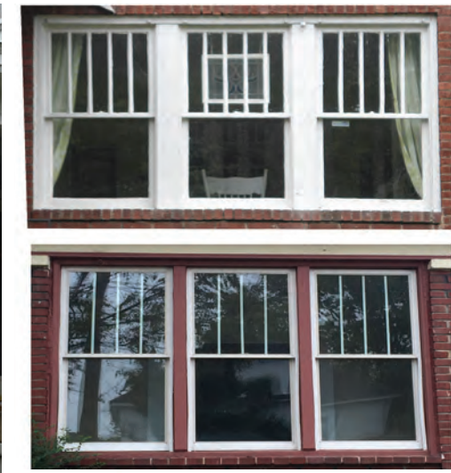
Top: Original Windows with True Divided Lights Bottom: Replacement Windows with Snap-in Muntins
