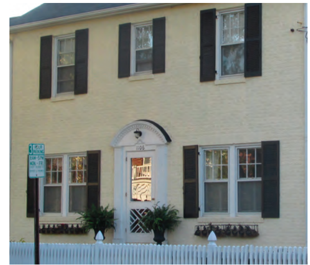
Centered Windows and Entrance with Chippendale Pattern Storm Door
