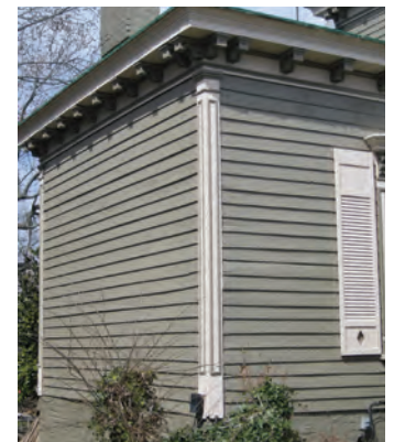
Italianate Bracketed Cornice
