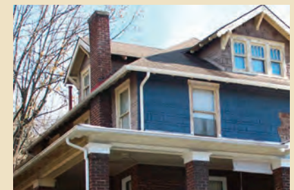
Example of architecture and integrated hidden gutter system
