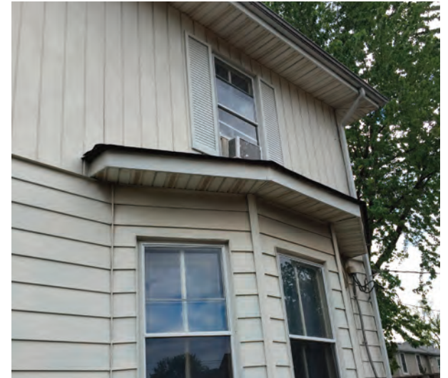
Horizontal and Vertical Siding Covers Walls, Window Trim, and Soffits
