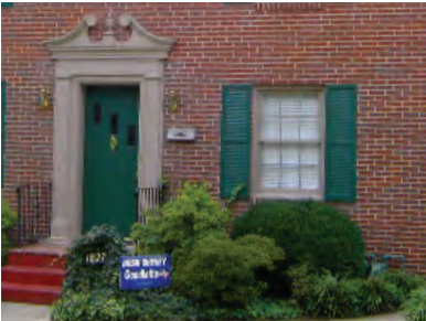
Prominent Entrance and Windows with Shutters
