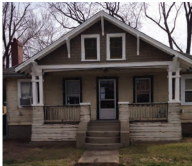
After: Removed siding, features uncovered and restored
