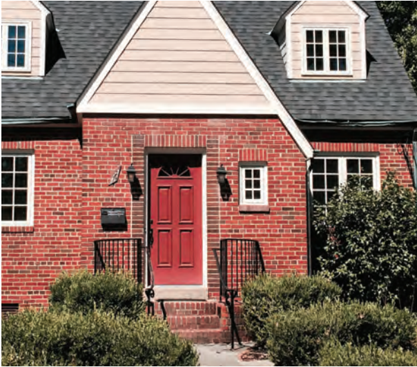
Soldier Course Brick over Window and Door
