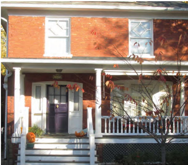
Tapered Columns, Turned Balustrade
