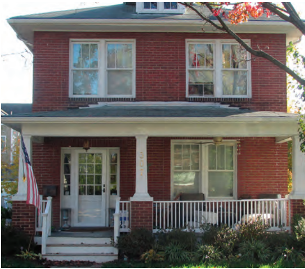
Wood Columns on Brick Piers, Paired Windows
