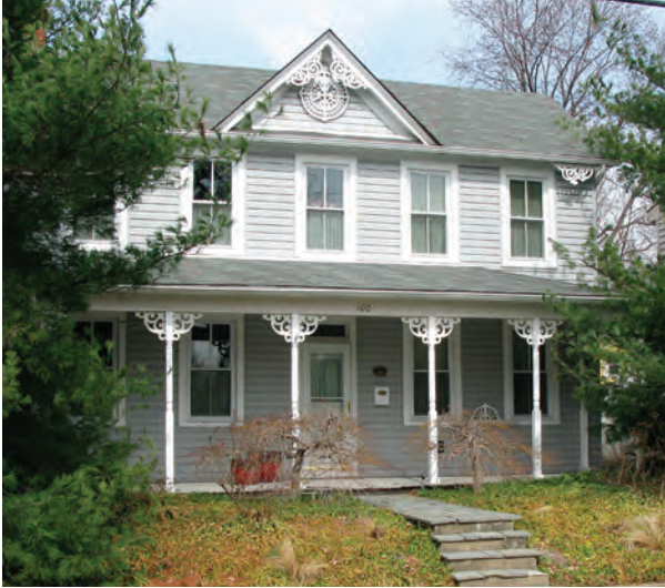
Two over Two Windows and Decorative Gable Vent
