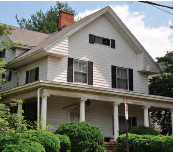
Eave Returns Covered with Siding
