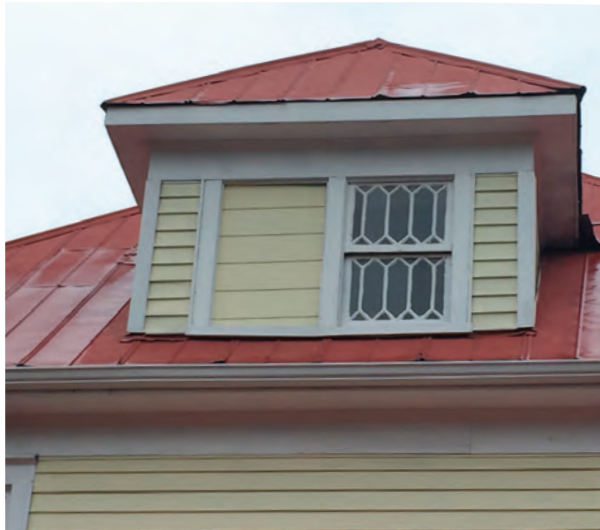
Decorative Dormer Window Removed and Replaced with Siding
