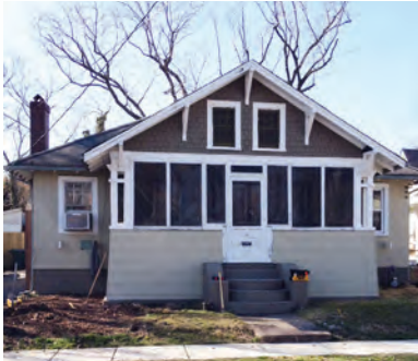
Before: Porch enclosed, siding covers front porch features
