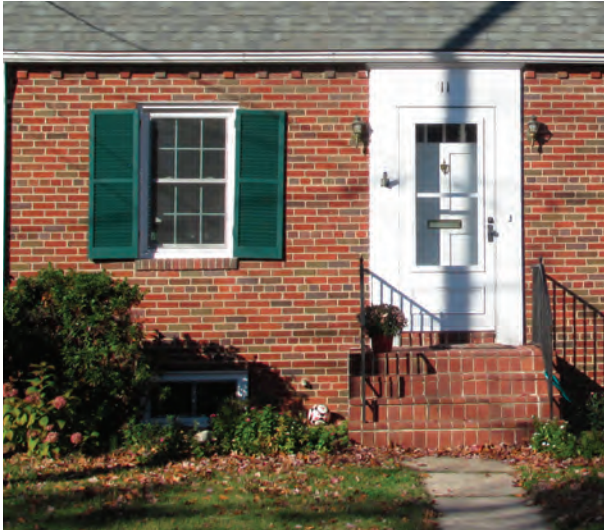
Brick Dentils at Cornice
