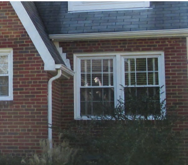
Six-Over-Six Paired Windows
