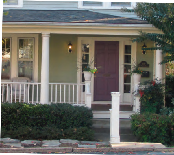
Doric Columns, Door with Sidelights
