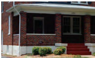
Brick Columns and Solid Railing
