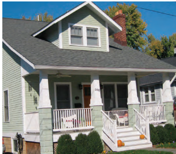
Masonry Piers with Tapered Wood Columns
