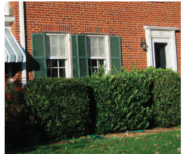
Soldier Course Brick Above Windows
