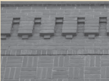
Brick corbelling on cornice
