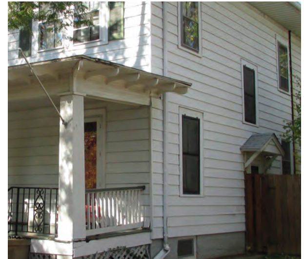
Tapered Columns and Exposed Rafters Front Porch
