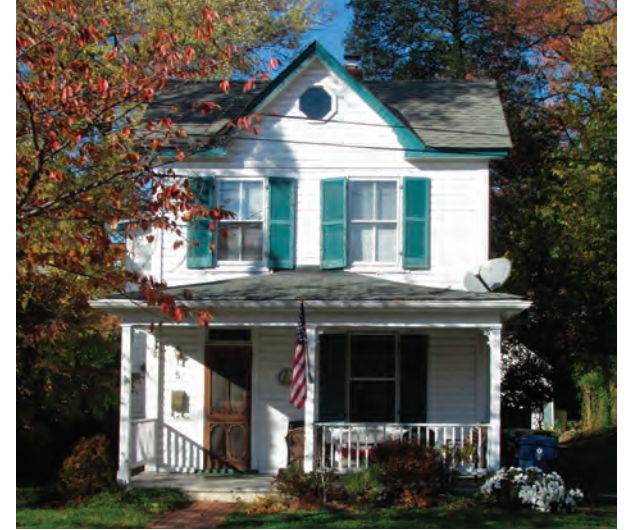
Octagonal Vent in Front Gable
